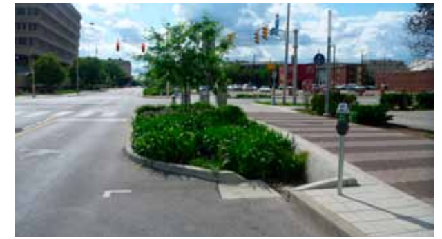
Stormwater Planter at Curb Bump-Out
