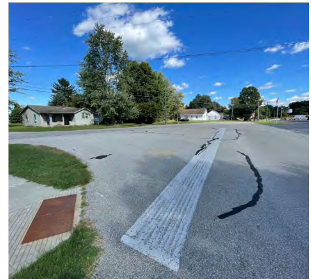
Existing Rullman & Main Intersection
