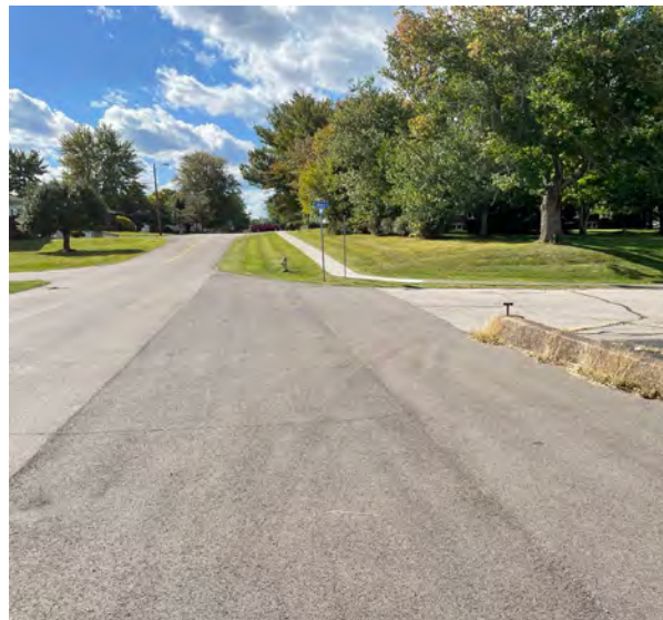
Existing Lenover & Miller Intersection
